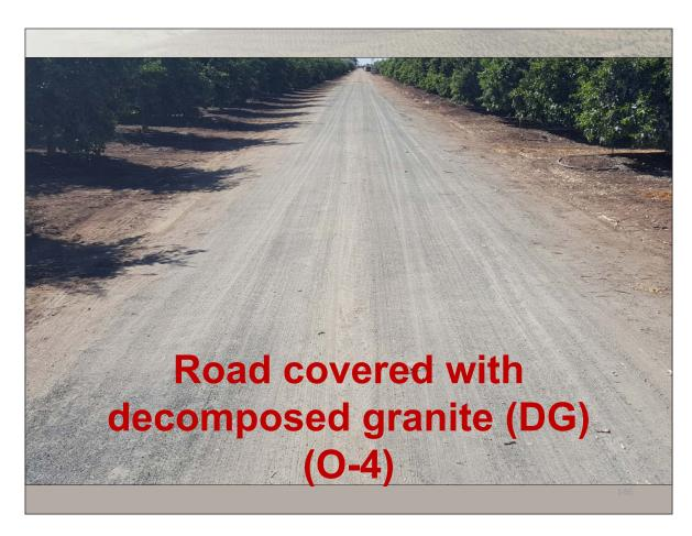
Covering the road with decomposed granite protects the road from the impact of rain drops. It is also less likely to erode because the particles are larger than soil particles. Decomposed granite is also porous, helping the water to infiltrate into the ground.
