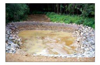
Operation and maintenance requirements will include periodic inspections with prompt repair or replacement of damaged components, periodic removal of sediment, and periodic mowing of vegetation.
