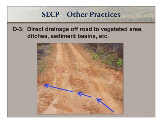
O-3: Direct drainage off road to vegetated area, ditches, sediment basins, etc.
