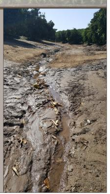
The gully can be seen on the side of the road. This gully is at a fairly steep hill, which means the water will be flowing fast.
