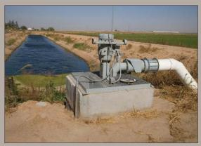
I-3: Recirculation systems are used to keep sediment and farm inputs on site. Water is recirculated to irrigate other fields.
