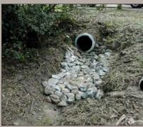
I-6: Use of flow dissipaters to minimize erosion at discharge point.
