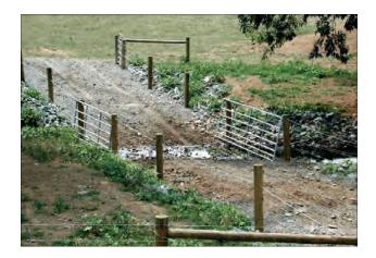
Evaluate the need for safety features such as guard rails and reflectors on culvert or bridge crossings, and water-depth signage on ford crossings.
