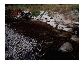
This practice has a minimum expected life of 20 years. Operation and maintenance requirements will be specific to the type of treatments selected for the site. The site must be inspected periodically and after storm events. Vegetation may have to be planted multiple times to ensure good establishment. Structural measures, such as riprap or gabions, may need to be repaired or replaced.
