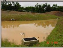
I-15: Sediment basins / holding ponds are used to settle out sediment and hydrophobic pesticides such as pyrethroids from irrigation and storm runoff.
