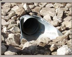
All culverts should be checked regularly and cleaned when necessary. Water often discharges from culverts at a higher velocity than the soil downstream can handle. Riprap should be placed downstream of the culvert to protect the soil from erosion.
