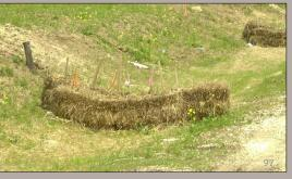
Straw bales intercept and catch sediment suspended in runoff. Generally a temporary measure that requires routine maintenance. They must be probably installed and staked into the ground. Poor installation can result in greater erosion issues.
