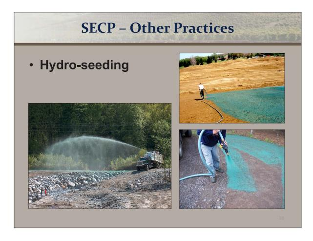
Hydroseeding is a planting process that uses a slurry of seed and mulch. The vegetation that is grown here can be used to trap sediment and aid in settling prior to discharging off of the parcel. Not that common in agriculture in the Central Valley. May have to irrigate. Hydroseeding is especially helpful at establishing vegetation on steeper slopes.
