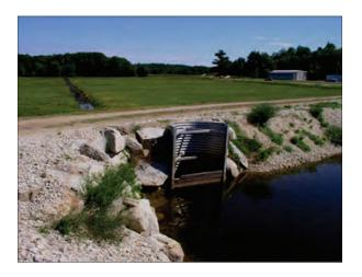
facility will depend upon the type of system chosen by the operator. The operation and maintenance plan will describe the amount and timing of water level management needed for the planned system. Semiannual maintenance will include inspection of the components and removal of debris. Additional inspection will be needed after major storm events.
