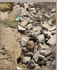
The roadside gully formed because the water velocity increased as the hill steepened. Gravel in the existing gully will protect the gully from eroding further. Riprap at the start of the downslope will help to dissipate excess energy as water begins to flow downhill. Other practices could be used, such as grassed waterways. Determine the potential recommendations that make the most sense for your farm, field, topography, climate, etc. Each SECP is intended to be custom-fit to the farm.
